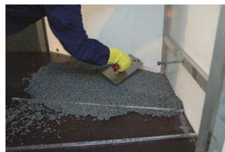
6. Application of 1 mixing unit of app. 6 kg
