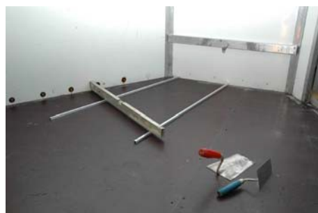
5. Extra needed material: ledges, trowel, waterscale
