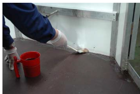
3. Pre-Treating of joints with primer 1103
