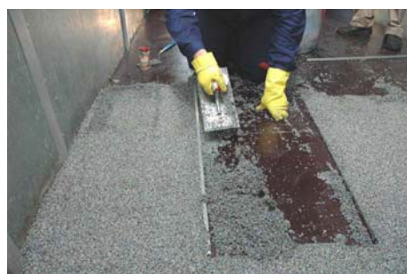
7. work Step by Step towards the exit ...
